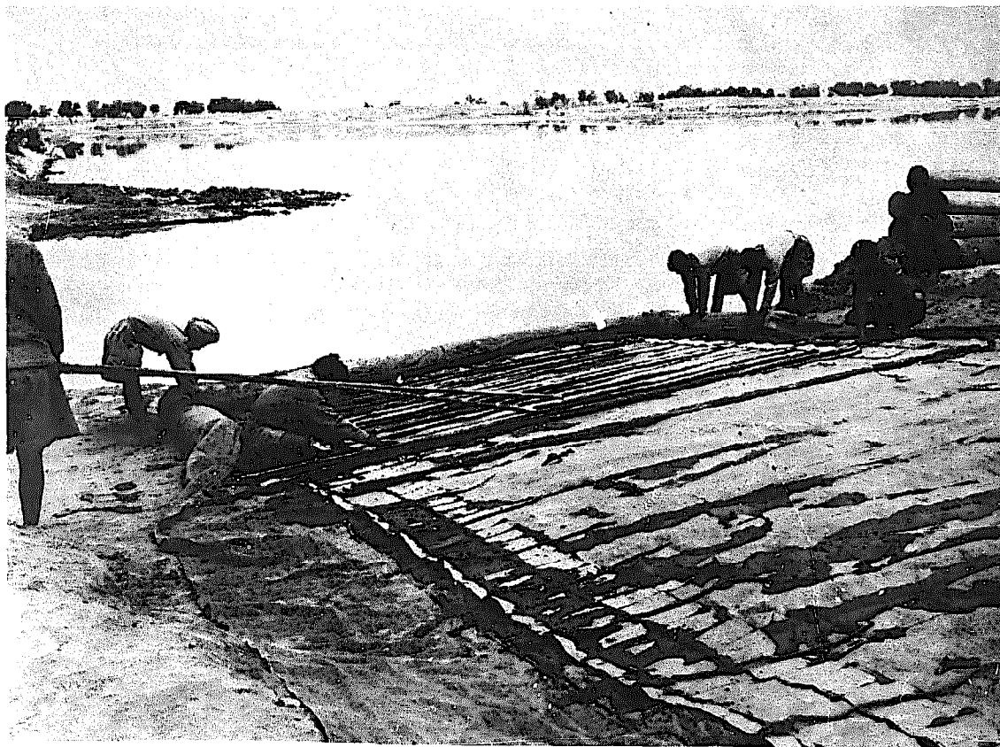
Photo 1. Bamboo inserted into the matbridge.
