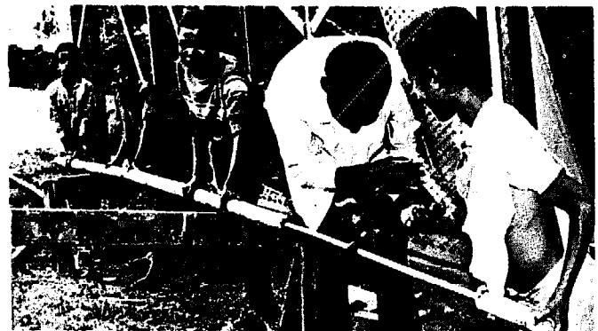
2. The drilling operation
